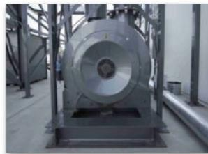
At the heart of each of our central vacuum systems are our powerful, continuous duty, multi-stage, centrifugal fans. Offered on 3 different platforms and with up to 9 stages, these fans pro-
